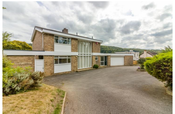
Garage 19'7" x 15'10" Integral double garage with electric up and over door, electric light and power, window to side and internal door to the entrance. This is accessed from a spacious curved coach circle type driveway with access at either end onto Sharp Lane and is surrounded by landscaped borders with mature shrubs.
