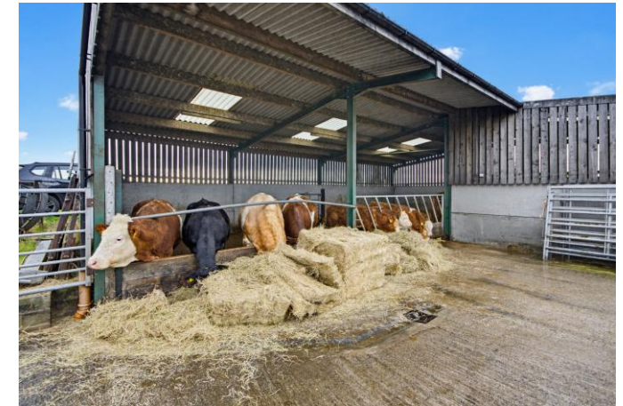
Building 2 48' x 19' plus 19'11" x 18'6" An additional L- shaped cattle shed.
