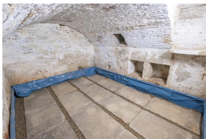
Cellar 3.61m x 2.82m A vaulted cellar with light and power sockets, flagged floor, stone storage recesses, air vent, and a capped off incoming gas pipe should you ever need a gas supply.
